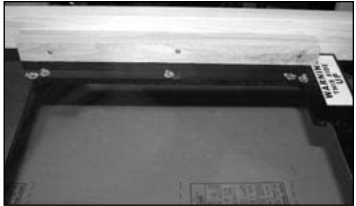
Figure 2: Overhead view of PIR, showing blocking attached to joist.
